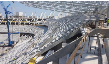
Prestressed grandstand elements.
