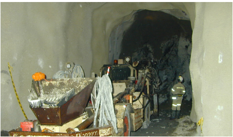
MSFR Shotcrete Ground Support.
